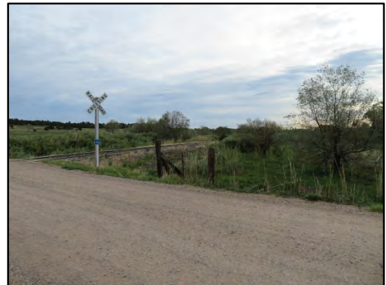
The Iowa Pacific rail line includes multiple crossings of county roads within the Study Area including a SH 12 crossing on the north side of La Veta.
