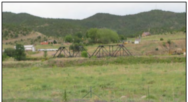
The original through-truss bridges over multiple crossings of the Purgatoire River can be seen from the Corridor.
