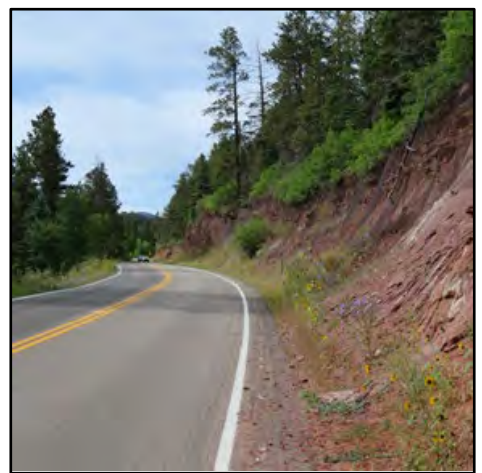
Typical narrow shoulder with rock debris, located between La Veta and Cuchara.
